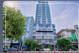
Ho Chi Minh, Vietnam Khai Hoan Building, District 11
